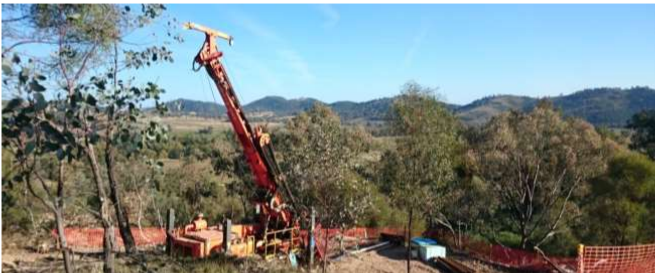
The diamond drill rig at Commonwealth South
